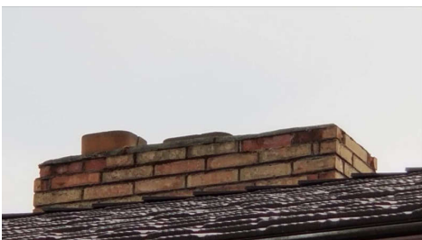
Cracked bricks
