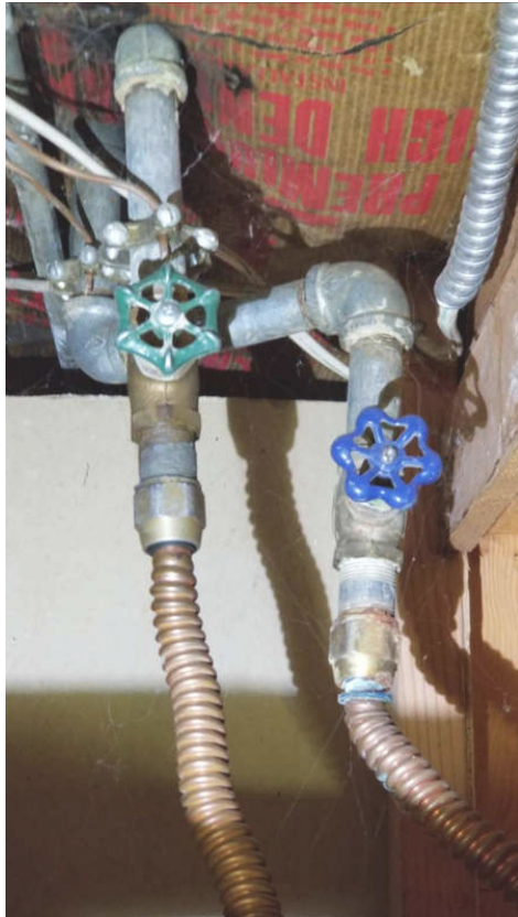
Basement water heater
