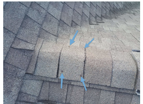
Exposed nail heads
