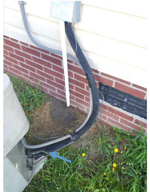
Damaged/ Deteriorated Insulation
