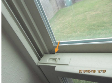
This window is off the railing.
