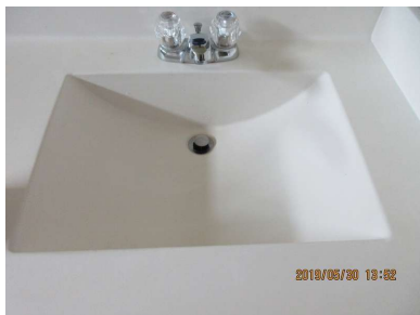
Sink upstairs between bedrooms is the primary drain for AC unit. It is constantly gurgling. Properly a venting issue. Recommend having a licensed plumber or HVAC professional evaluate.
