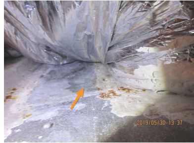
Moisture present on top of AC unit in attic with organic growth. Ductwork should not be laying on anything because it causes condensation which leads to moisture build up.
