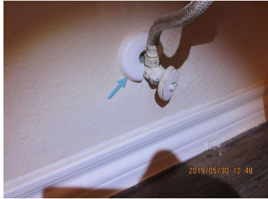
Esuceon not installed all the way.
