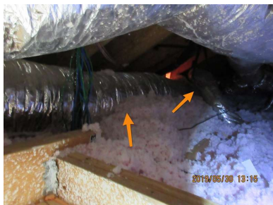
Insulation is laying on top and sides of much of ductwork in attic. Ductwork should not be touching insulation.
