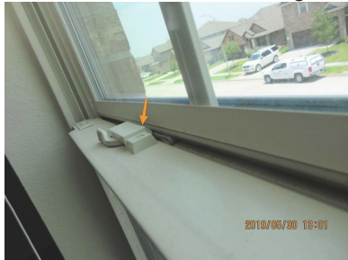
This window is off the railing.
