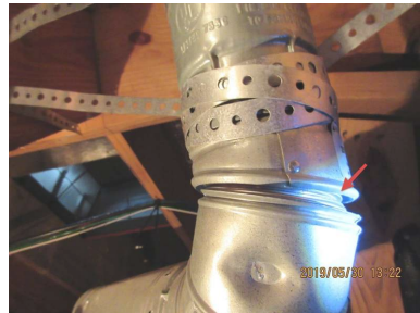
Broken flue.
