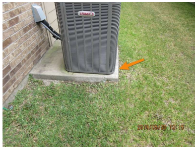
Recommend maintaining 3" exposed slab for unit.
