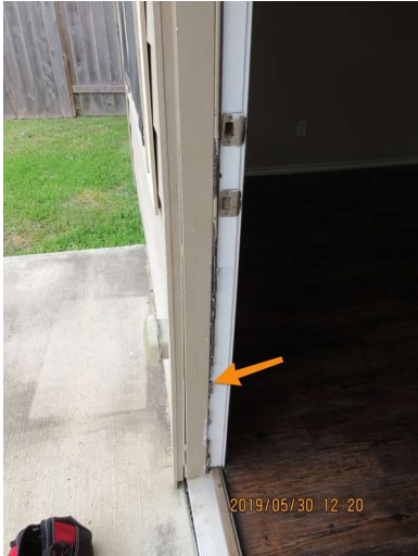
Weather stripping is damaged. Recommend replacing for proper sealing of house.
