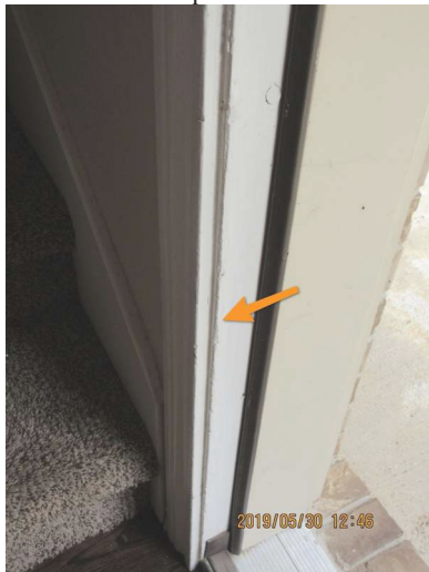
Poor workmanship. Cosmetic only.
