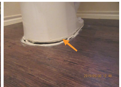
Recommend caulking around toilet. Toilet also appears to be lifted. This could be from using an incorrect toilet ring size. Recommend having a licensed plumber come out and evaluate.
