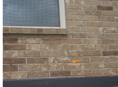
Cracked brick. See comments in "Foundations"
