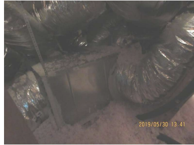
This plenum is resting in insulation. Which could be causing condensation to drip down to the laundry room below. Recommend having a licensed HVAC professional evaluate the entire ductwork and HVAC system for efficiency and proper installation of ductwork.
