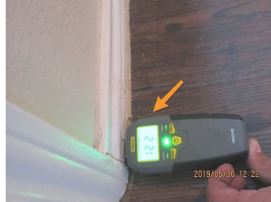
Right side (looking out) of back door. Visible moisture present. This is most likely due to the wood rot around the door not the exterior along with the siding not being 2" above concrete. Recommend removing and seeing what is behind the wood for any further moisture damage.
