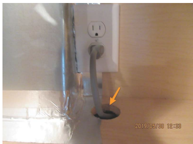
Exhaust should not be coming out of electrical hole.
