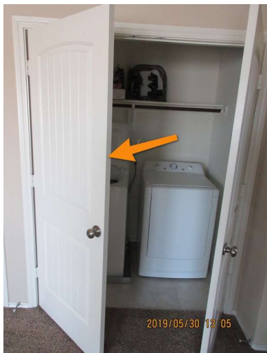
This door closes with out pushing it.
