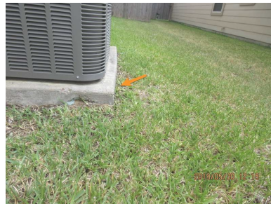
Recommend maintaining 3" exposed slab for unit.
