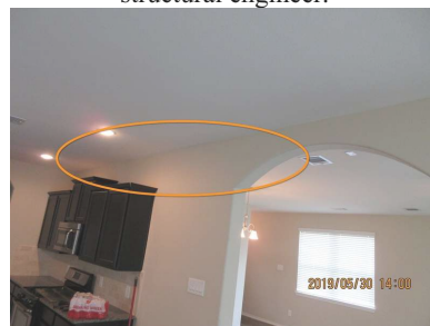
Crack starting to form on ceiling/wall joint. Recommend monitoring for future expansion of crack. This along with comments made in foundations section, recommend evaluation by structural engineer
