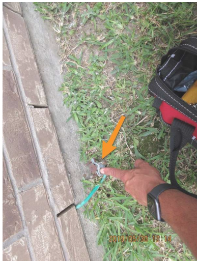
Ground wire clamp loose.
