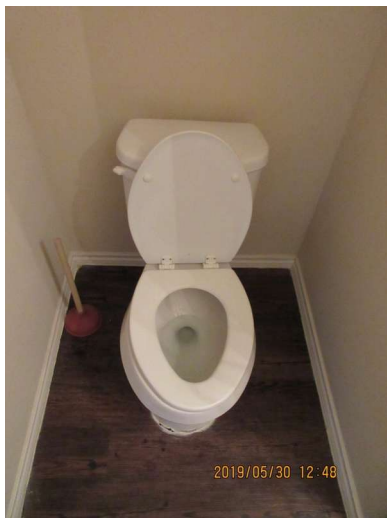
Toilet did not flush when handle was pressed all the way.
