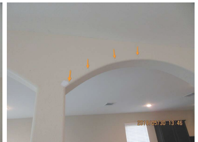
Repairs above arches. Recommend finishing repairs.
