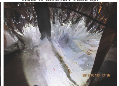
Moisture present on top of AC unit in attic with organic growth. Ductwork should not be laying on anything because it causes condensation which leads to moisture build up.
