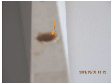
Top of laundry door. missing latch. Recommend replacing.
