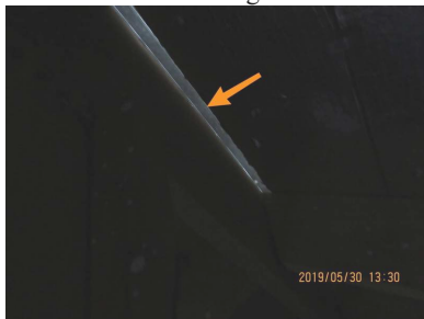
Extent of ridge vent.
