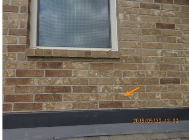
Cracked brick. See comments in "Foundations"
