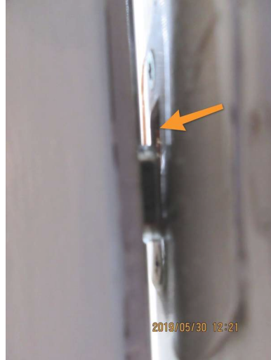
This shows distance that door is off.
