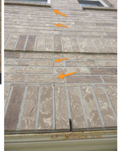
Cracked brick. See comments in "Foundations"
