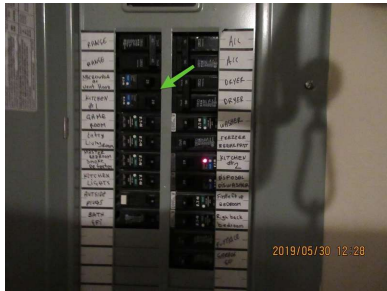
Vent hood fuse was blown at time of inspection.
