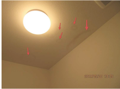
I believe this to be from the ductwork above the laundry room.
