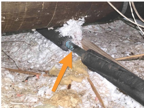
Condensation Inside Attic
