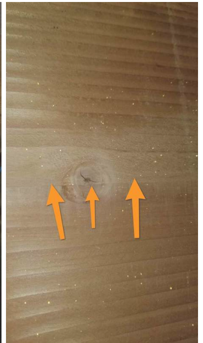
Above Garage Attic Hatch
