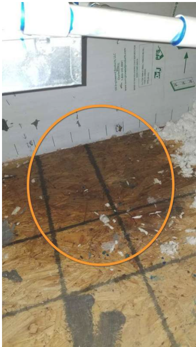
Area of Moisture
