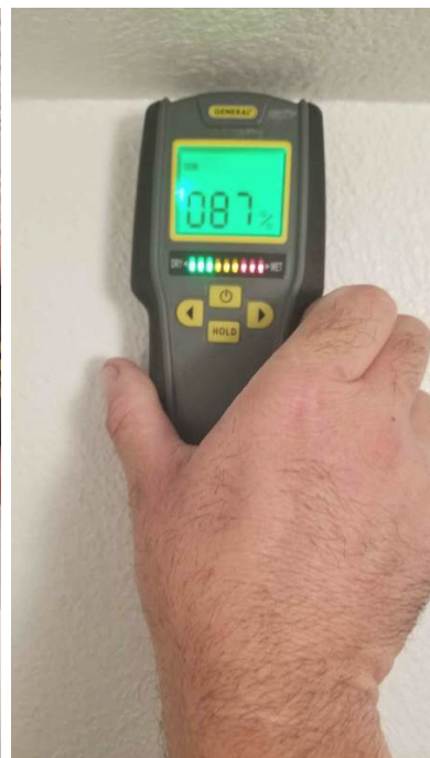
High Moisture Level , 2nd Floor Closet Wall
