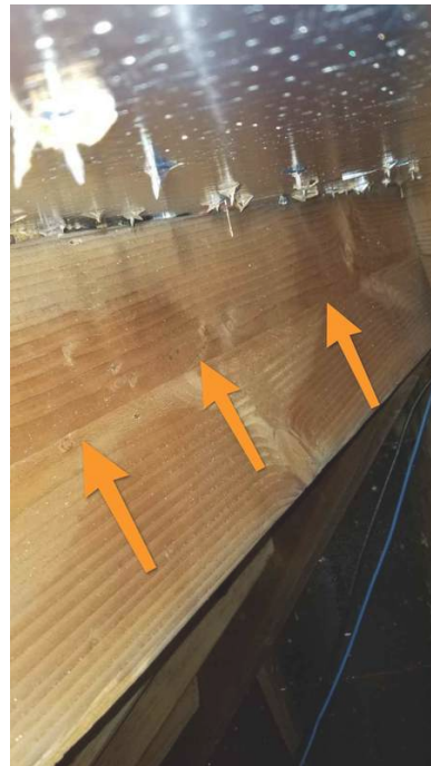
Above Garage Attic Hatch
