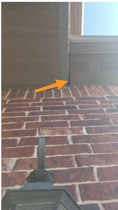
Above Front Porch, Exterior View
