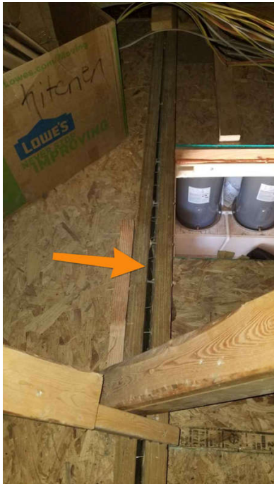
Attic Above Garage
