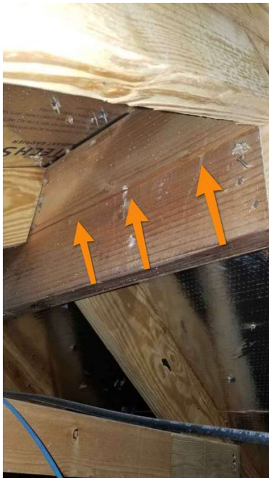
Above Garage Attic Hatch
