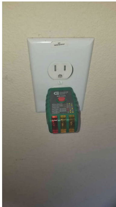
Garage Near Door
