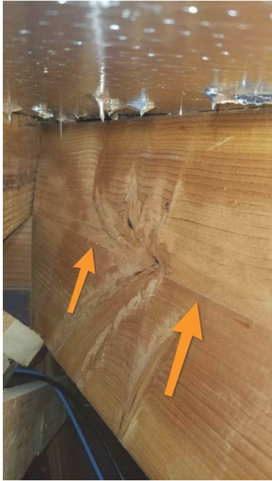
Above Garage Attic Hatch
