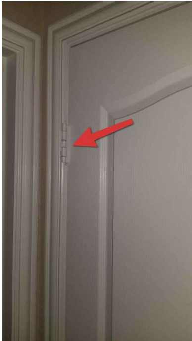
Door Leading to Garage Needs Self-closing Hinge
