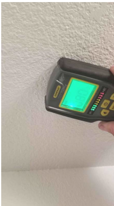
High Moisture, 2nd Floor Closet Ceiling
