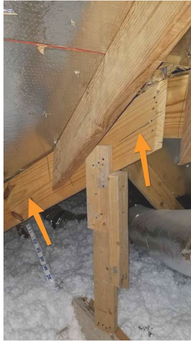
Attic Above Master Bedroom
