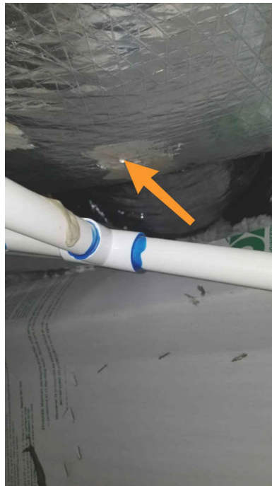
Dripping From Here
