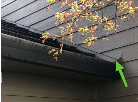
Kickout Flashing - Good
