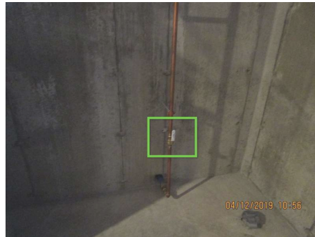
Main water shut-off valve
