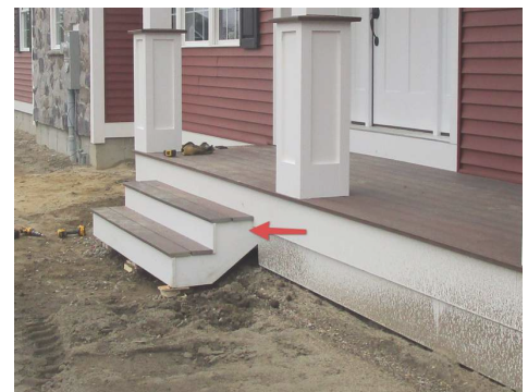
Steps were removed during inspection. Front Steps
