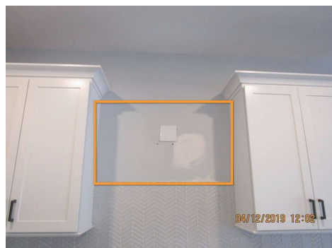
Kitchen-Exhaust hood missing
