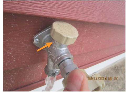
Leak observed at hose bib
