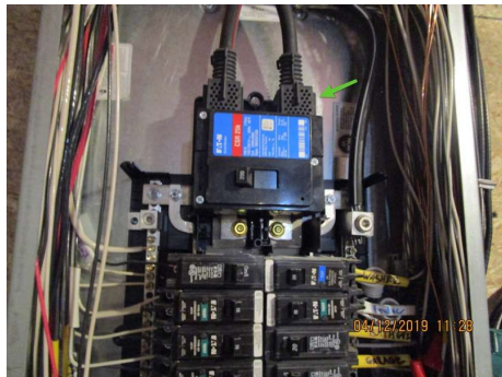
Service entrance cables have protected coverings. Connection concealed.
