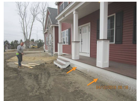
Front Porch underside concealed
