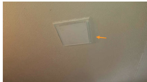
1st Floor Bathroom
