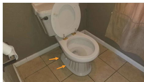
1st Floor Bathroom
