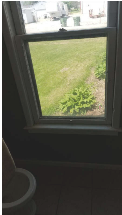
1st Floor Bathroom
