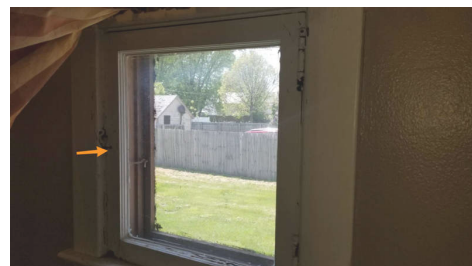
Kitchen behind fridge location
