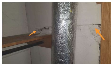
Dining Room closet under stairs
