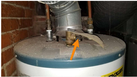
DISCHARGE PIPE ON TPR VALVE
