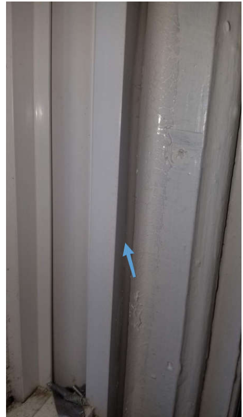
Majority of vinyl windows in home
