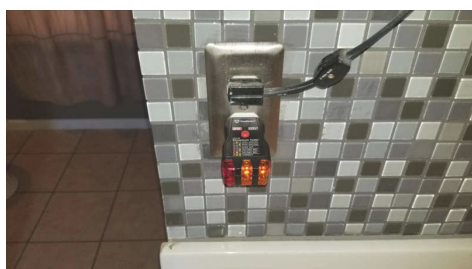
1st Floor Bathroom
