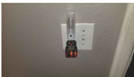
1st Floor Bathroom
