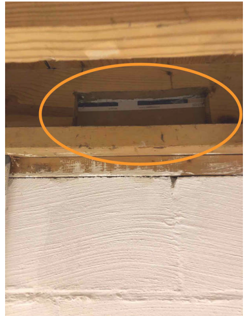
Northwest work room North wall
