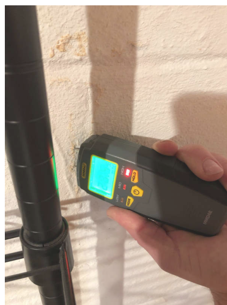
Northeast storage room
