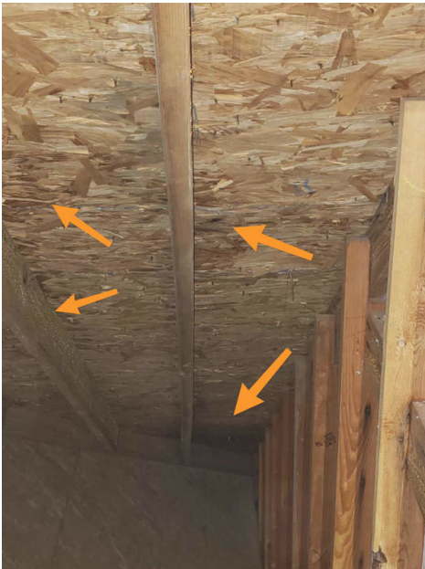
From attic facing front, Right corner lower attic area
