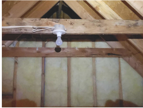
Attic Above Garage
