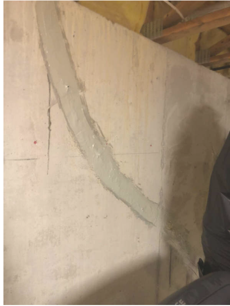
Basement Back Right Corner
