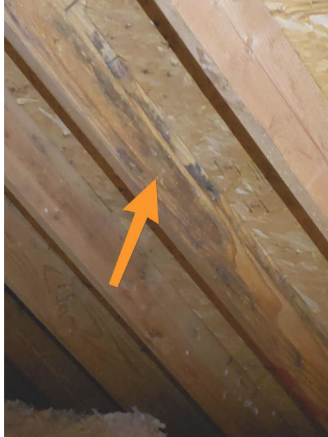
Attic Above Master Closet
