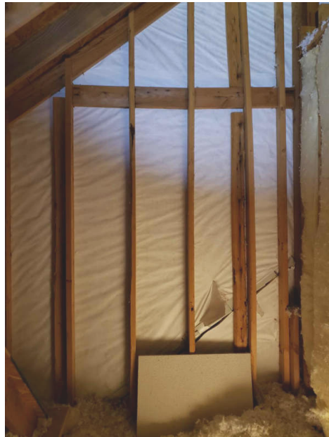
Attic Above Master Closet
