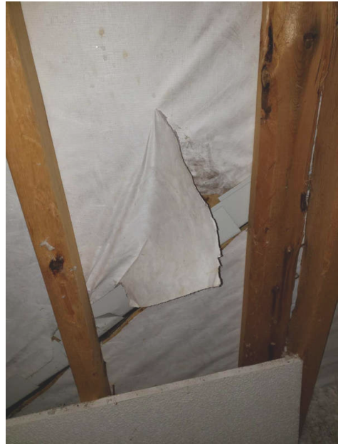
Attic Above Master Closet
