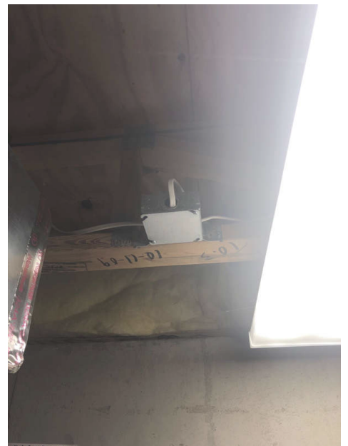
Basement Left Side Middle
