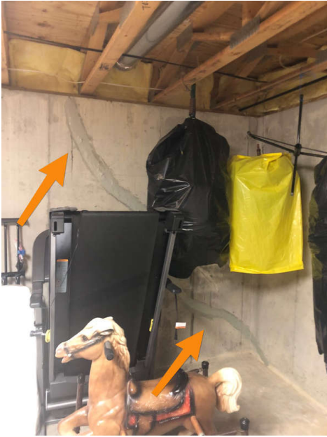
Basement Back Right Corner
