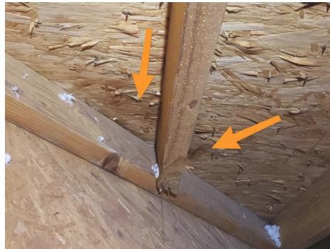
Attic Above Master Closet
