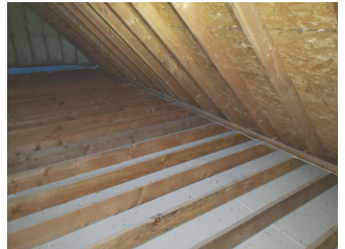
Attic Above Garage
