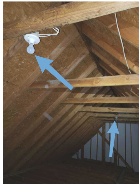
Attic Above Garage
