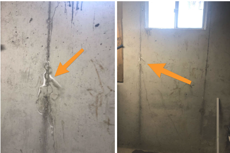
Front Right Corner
