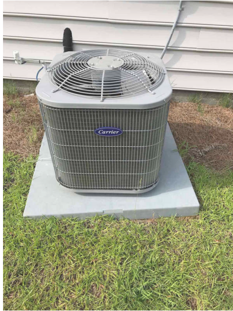
Heat Pump which also functions with AC
