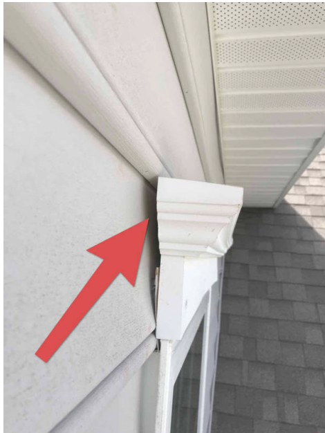
Trim above window in left elevation had an area where water can get trapped. Recommend window repair man review
