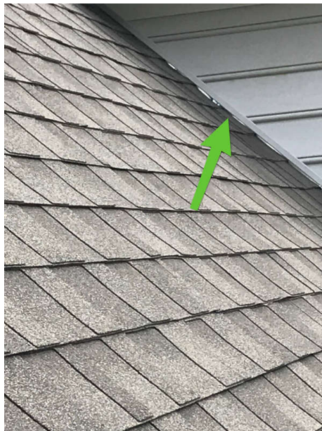
Flashing has been installed for single intersects siding
