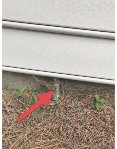
Tree growing under siding
