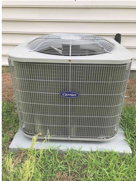
Carrier heat pump for upstairs is a 1.5 ton system
