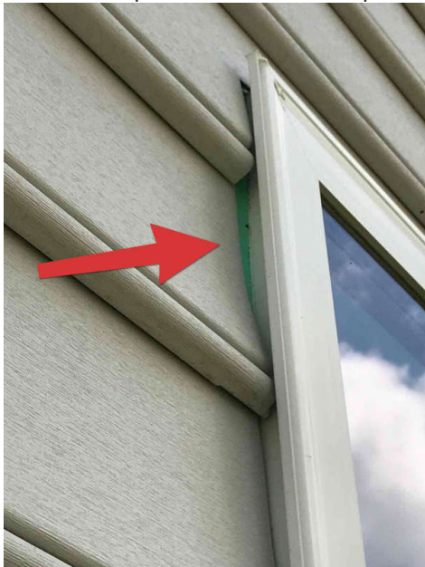
Sealant needed around exterior if windows or the windows are not properly flashed or trimmed
