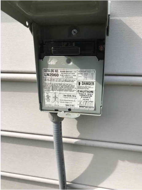
Pull disconnect rated at 60 amps is located above the heat pump
