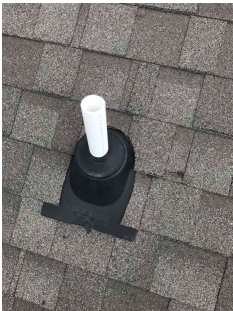
Overview of pipe jack flashing material.
