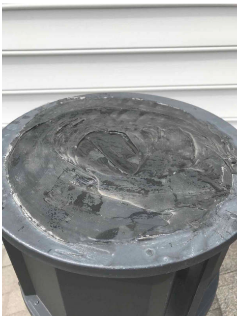
Chimney flue vents had a soft sealant applied to the top of it. Overview of flue with sealant over it.
