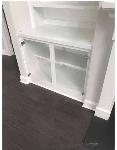
Cabinet Door are Missing in Living Room
