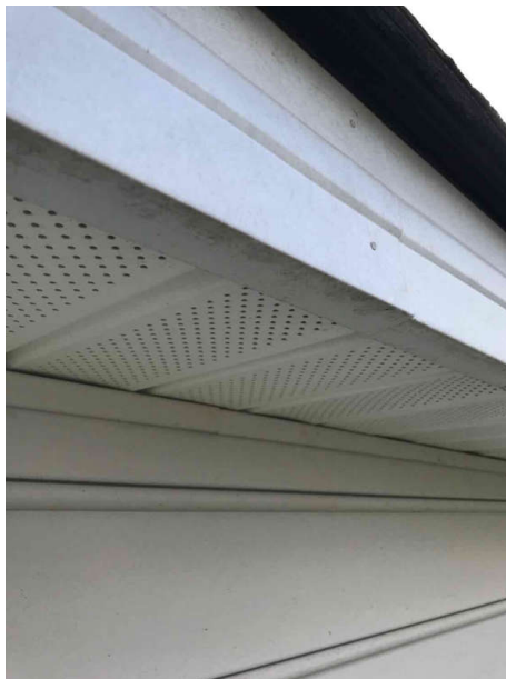
Vinyl vented soffit with metal fascia
