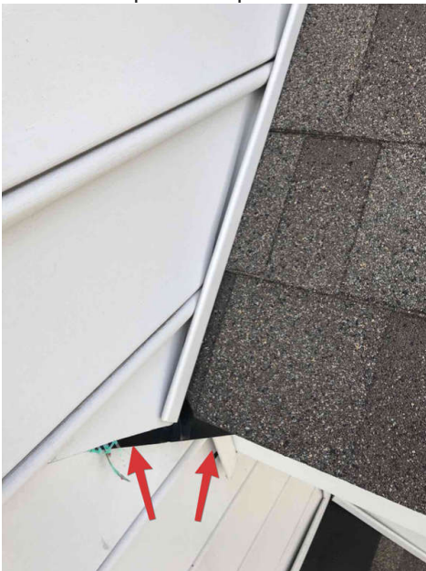
Cut in siding
