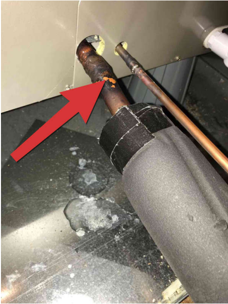
Water in pan from leaking copper. Piping
