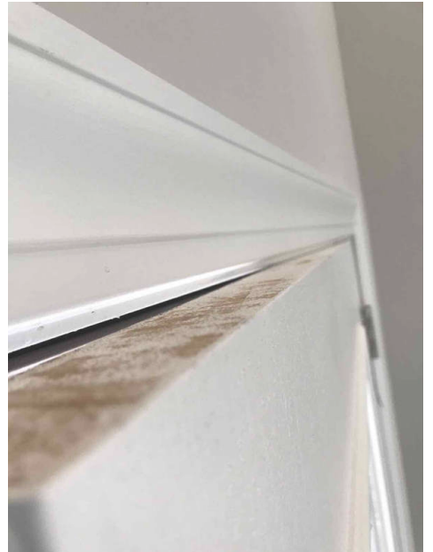
The top of the door has been shaved once
