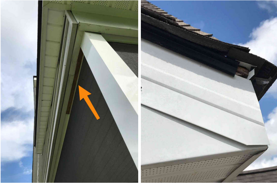
Bare wood needs to be covered with flashing
