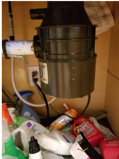
Garbage Disposal: Installed
