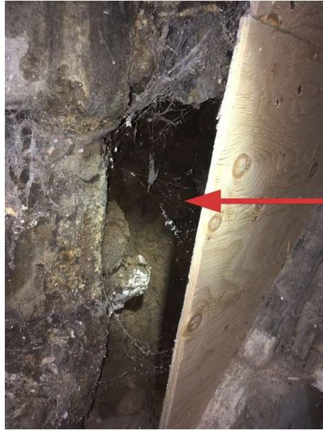
side of stairs; no able to check other side of stairs due to inaccessibility
