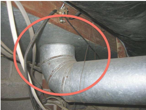
Loose connection; recommend sealing.
