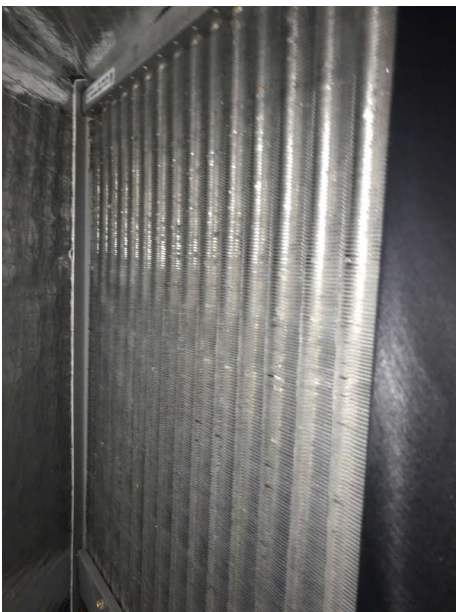
Coils are in great shape
