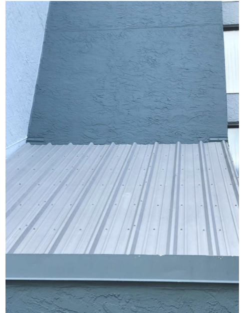
South, Missing Headwall Flashing
