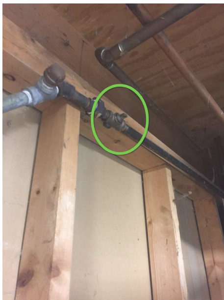
Gas Shutoff located above water heater.
