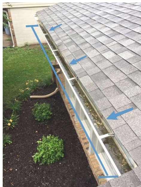
Approximately two inches of standing water in gutter.
