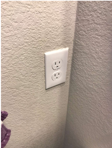
1st Floor Office Bathroom
