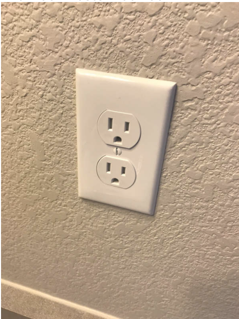
2nd Floor East Bathroom
