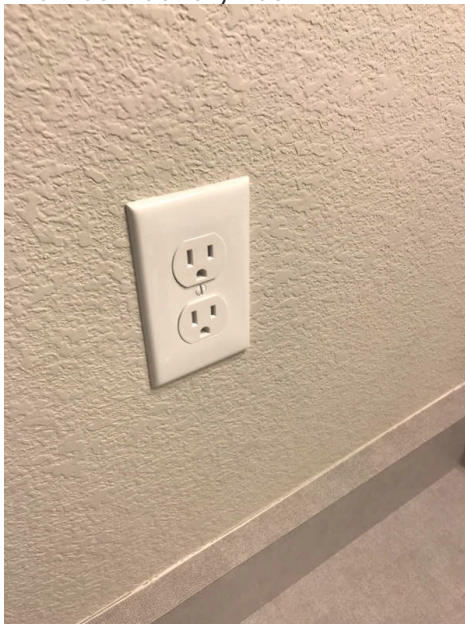
2nd Floor South Bathroom
