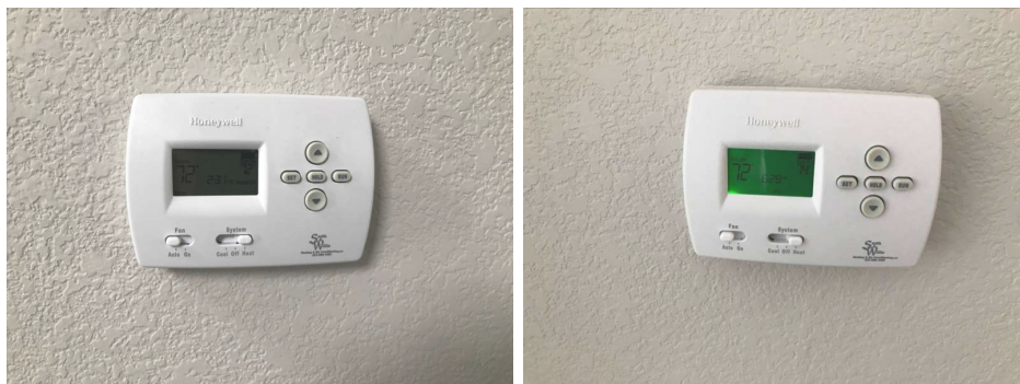
1st Floor Hallway
