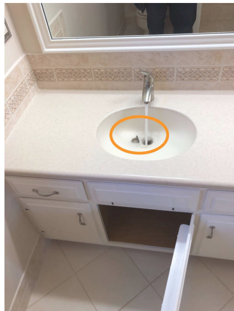
2nd Floor hall Bathroom
