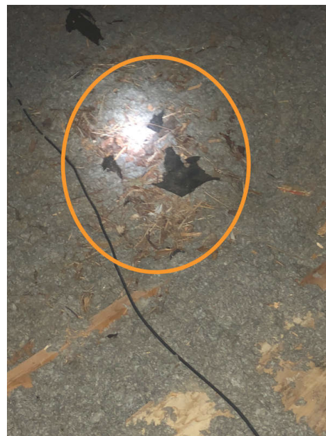
Attic near access
