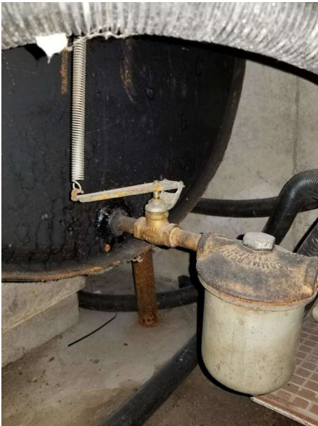
Location of Main Fuel Shut-Off At Tank
