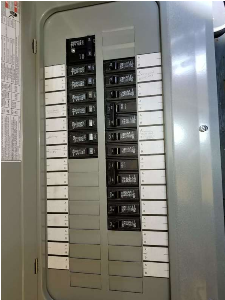
Location of Main Disconnect Top Bank
