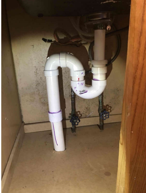
S-Trap vs. P-Trap
