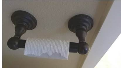
2nd Floor Bathroom - Right Side Loose
