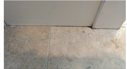
Master Bathroom - Needs Seal
