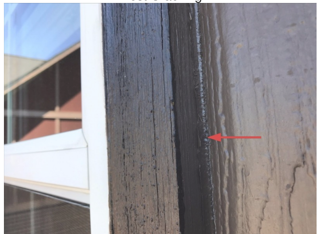
West - Needs resealing
