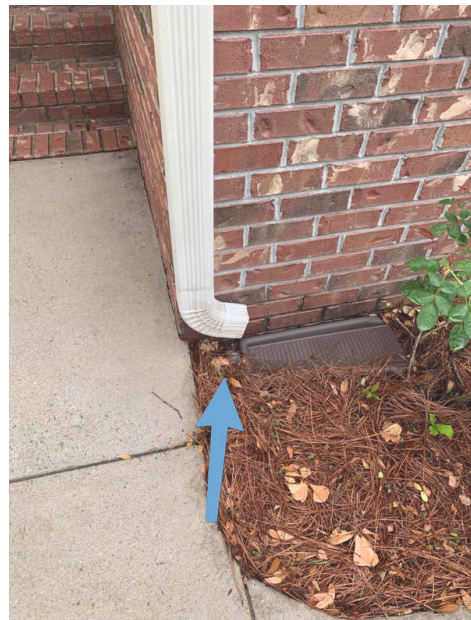
Front of the home
