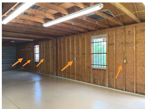
ALL receptacles in the detached garage
