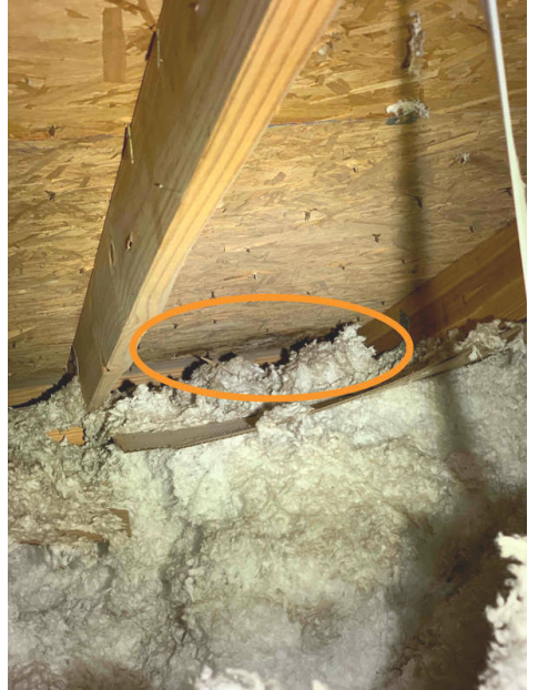
Front left corner of attic/ home
