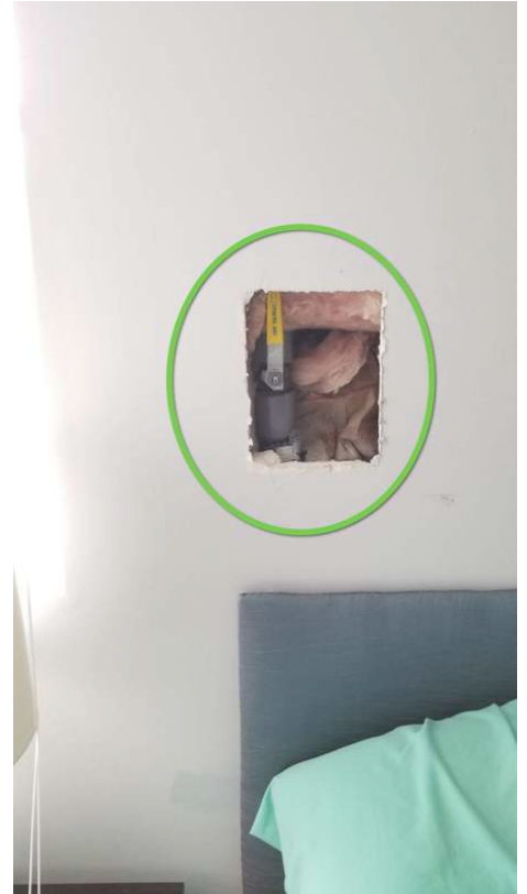
Water main shut off valve
