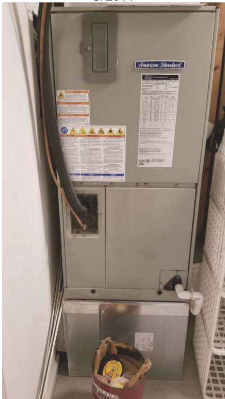
HVAC Central AC unit American Standard Model # 4TEC3F36B1000AA Mfg Date = 12/2010
