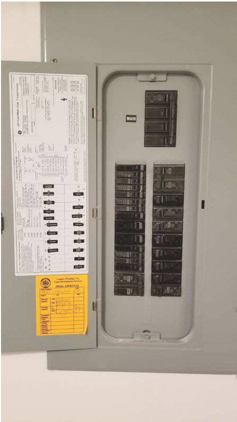
GE 200 Amp Circuit Breaker Panel
