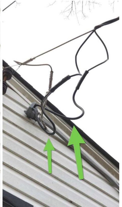
Service mast drip loop present
