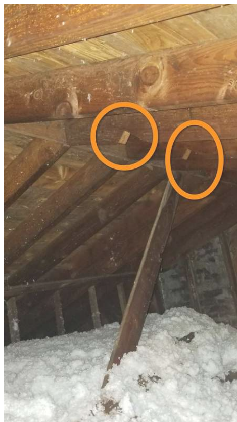
Notches cut out of rafters
