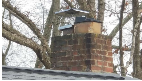
Exterior chimney crown with chimney cap
