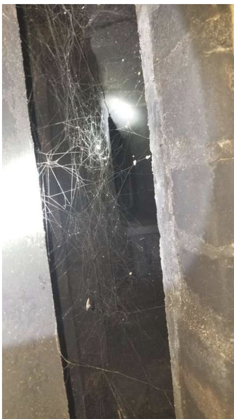
Visual of Inside the firebox and flue pipe. Recommend a level 2 chimney inspection to determine condition of flue pipe
