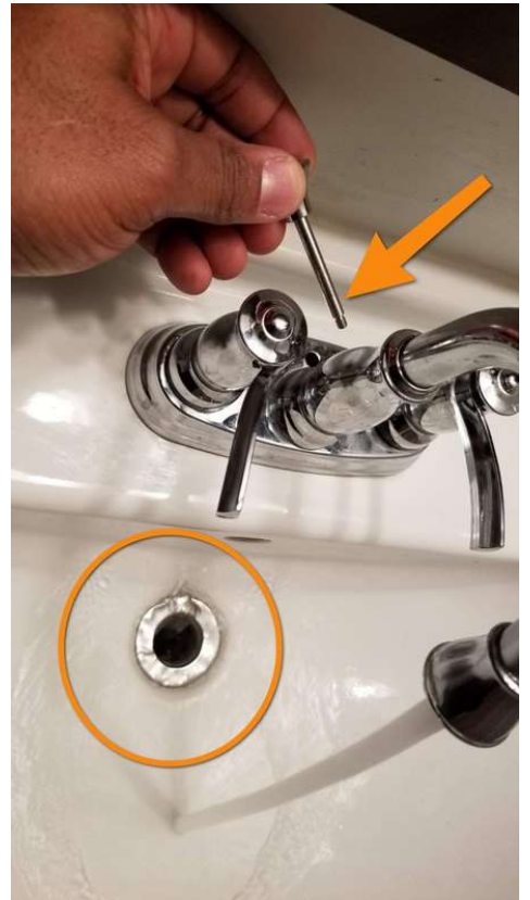
Stopper missing and broken
