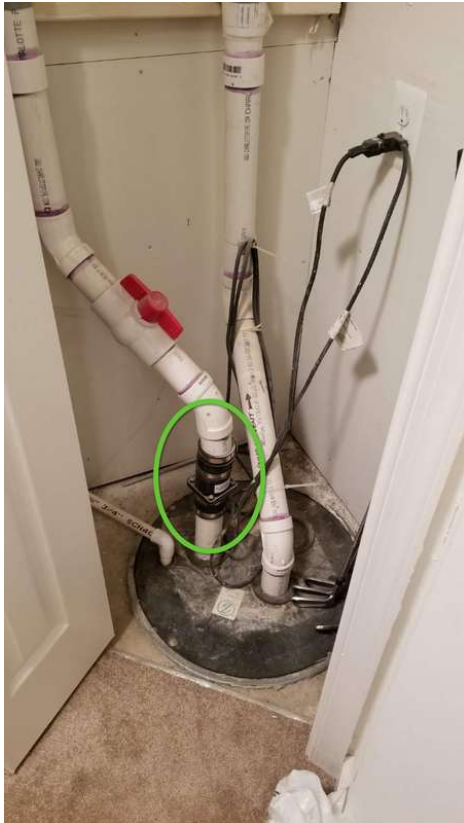
Green circle= Check valve installed
