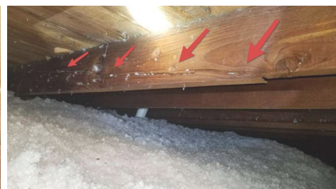
Rafter is splitting very badly and needs to be evaluated by a roofing professional
