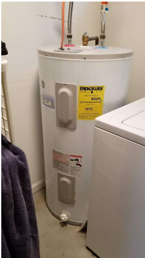
Hot water heater GE Model # GE50M06AAG MFG date = 5/2011 Capacity = 50 gals
