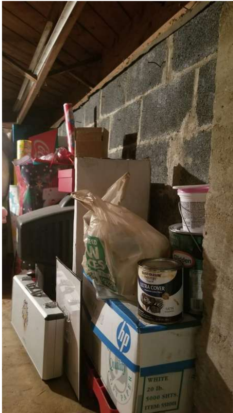
20% of foundation is masonry block
