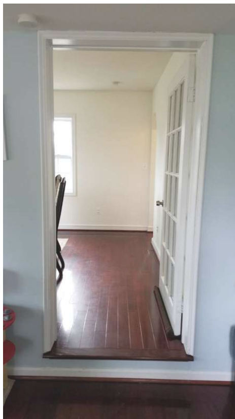
Door leading to the interior of the house
