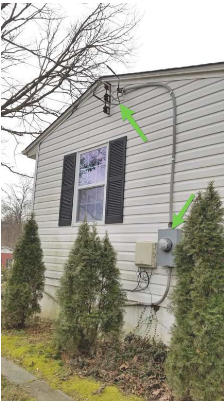
North frontside of house Electric Service Utility for house
