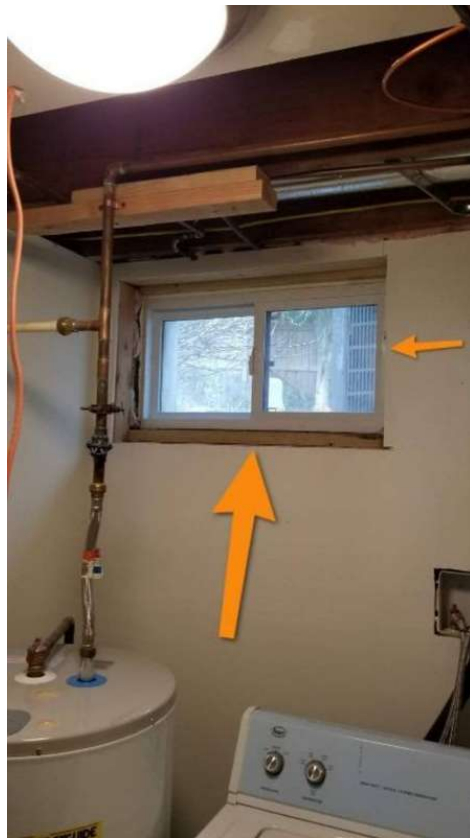
Laundry room window. Not an egress window
