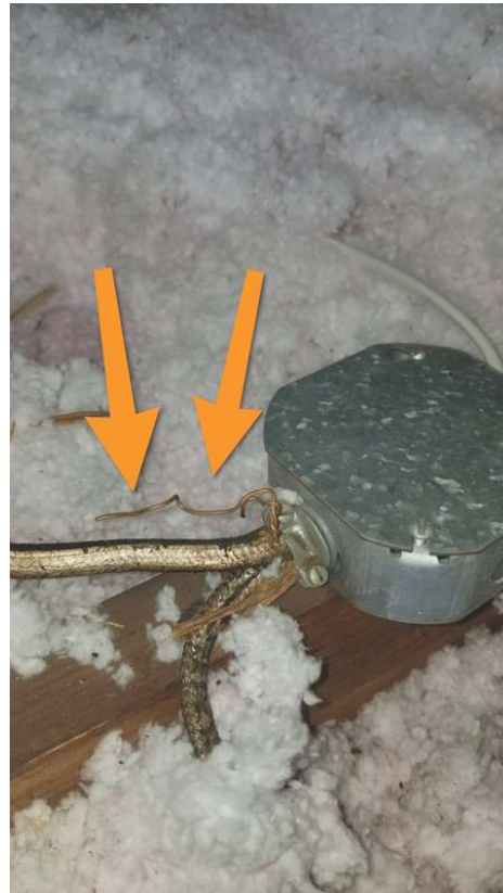
Possibly aluminum wiring in the attic leading to the Gabel attic fan needs to be evaluated further by a qualified licensed electrician
