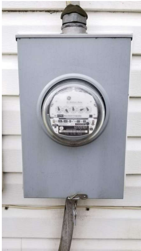
North front House Service Utility Meter
