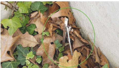
Westside of house Grounding rod
