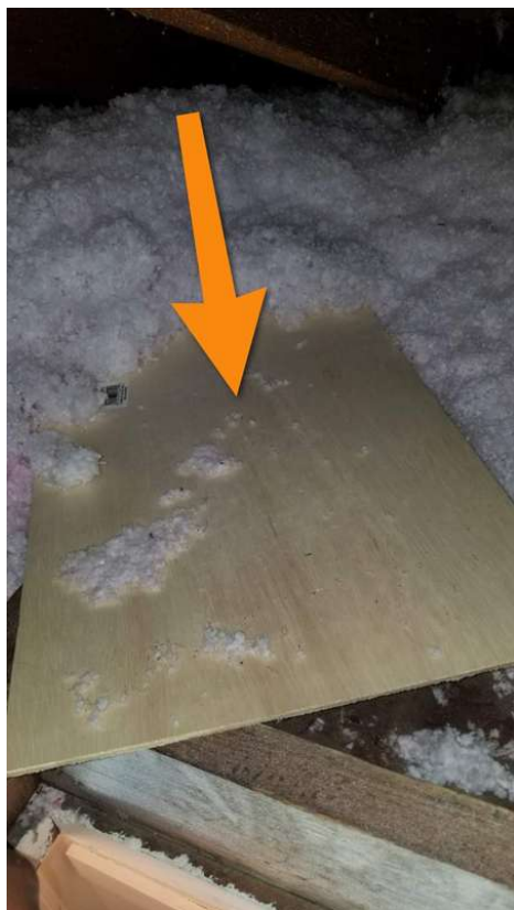
Lack of insulation around attic access door causes energy loss
