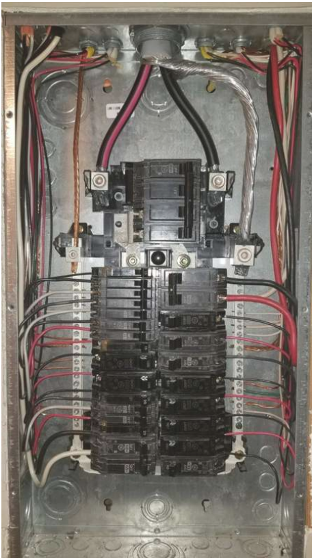
Circuit breaker panel with cover removed
