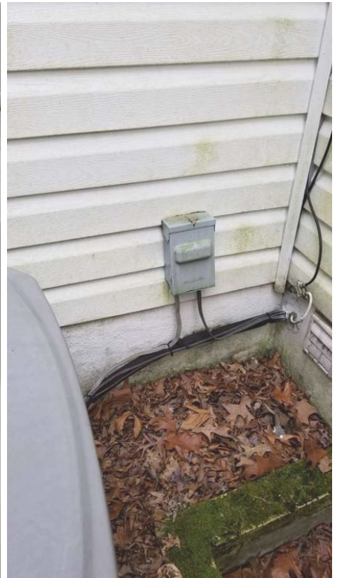
Condensing unit shut off breaker
