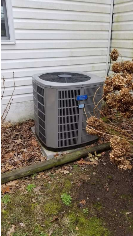
Outdoor Condensing Unit American Standard Heritage 13 Model # 4A6H3030B1000AA MFG Date = 5/2011
