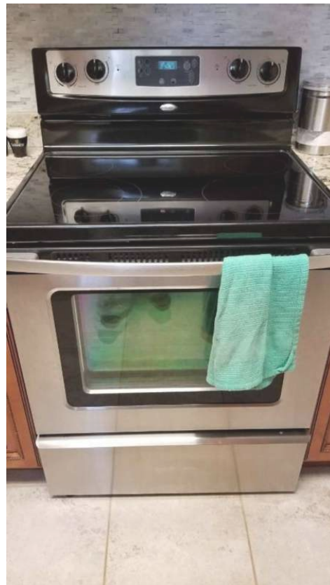
No anti tip attached to the range
