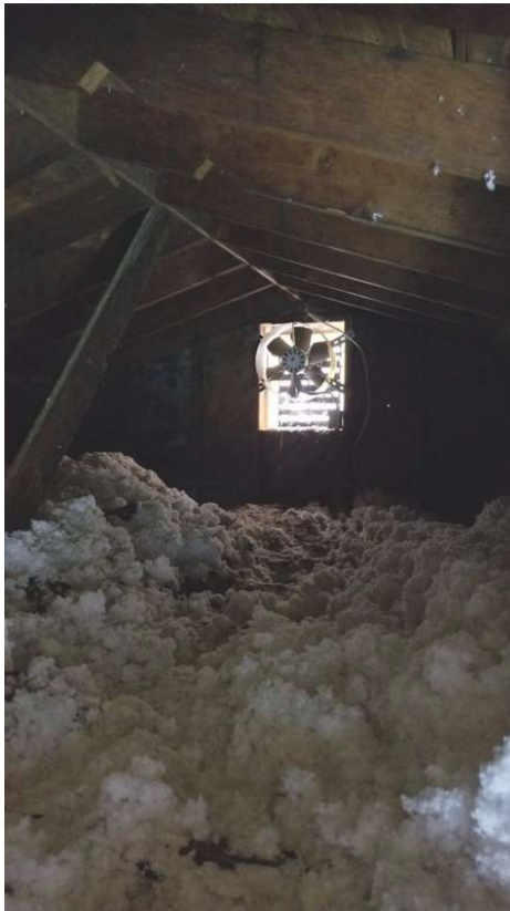
Gable attic fan observed but could not determine whether the unit was working. Recommend having a qualified electrician evaluate
