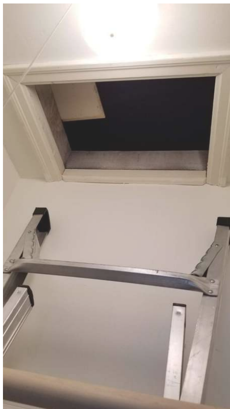
Attic entrance small
