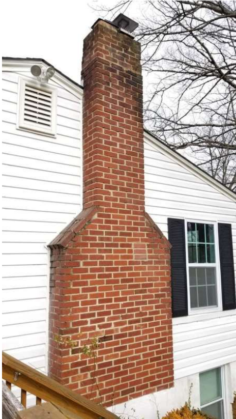
Exterior Brick Chimney
