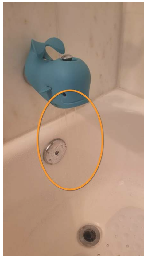
Water not properly diverting to the shower head
