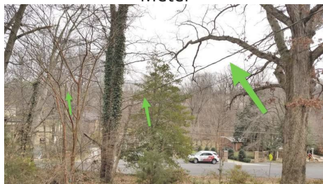
House service utility wires from the street
