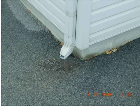
Gutter extension is sending water up hill.
