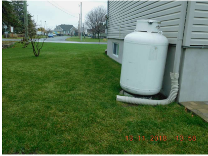
Gutter extension is sending water up hill.
