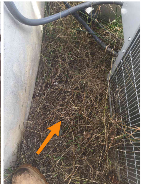
Rear of a/c unit
