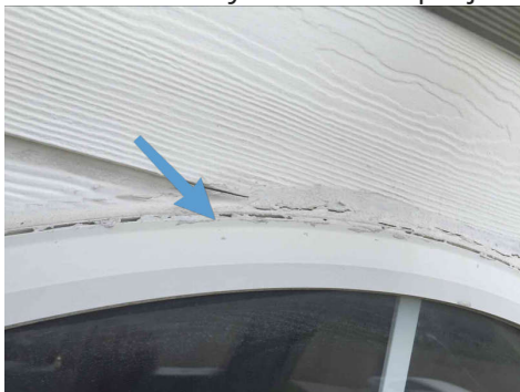
This area is excessively caulked. May be an indication of past water intrusion.
