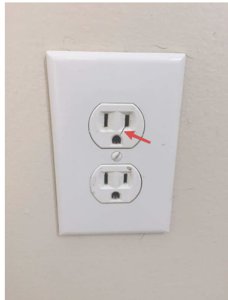
Crack may get worse with use
