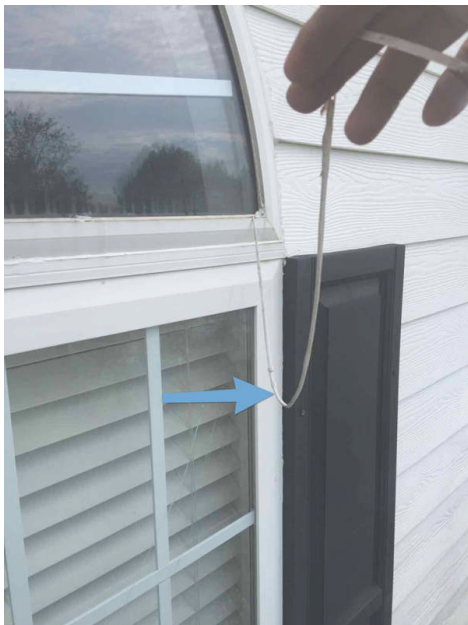
This area is excessively caulked. May be an indication of past water intrusion.
