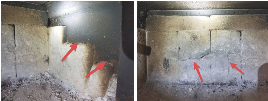
Damaged bricks
