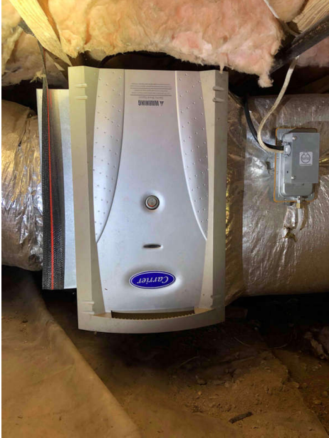
Air purifier system located in crawlspace for downstairs unit.
