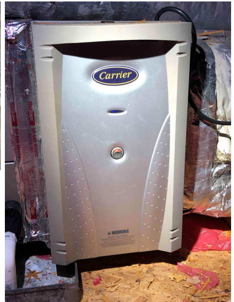
Air Purifier attached to upstairs air handler.
