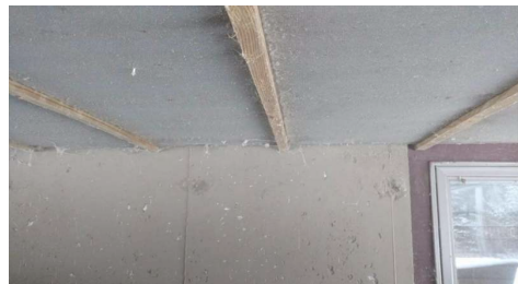
Underneath the back porch, when viewed with a flashlight the ledger was visible, but not able to be photographed.
