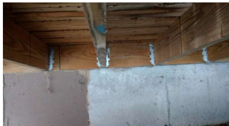
Underneath the front porch.
