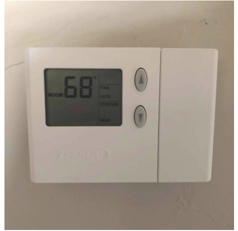
2nd Floor Hall
