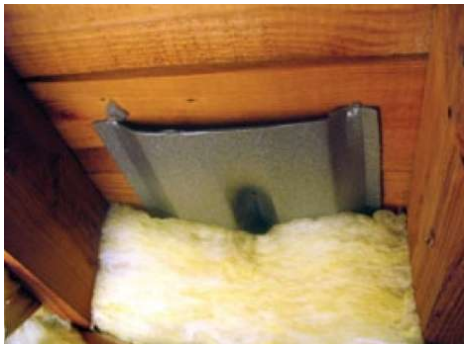
Insulation Baffles
