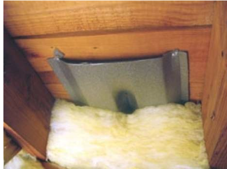
Properly Installed Insulation Baffles
