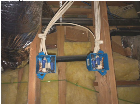
Basement utility room
