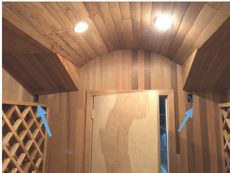
Basement wine cellar
