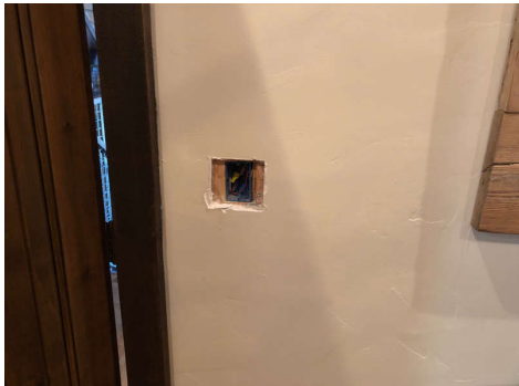
2nd Floor South Bedroom
