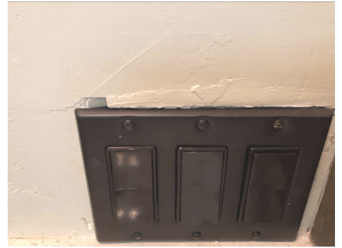
1st Floor Southwest Bathroom
