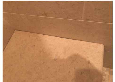
1st Floor Southeast Bathroom
