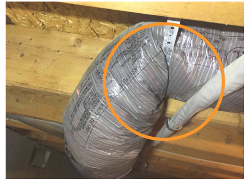
Restriction to airflow. Crawlspace
