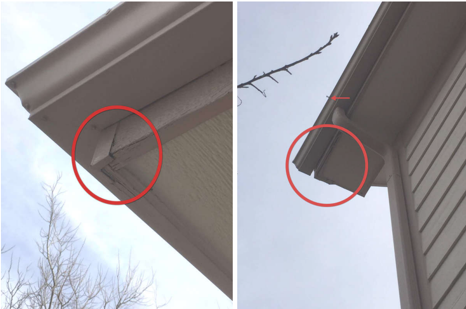
Minor cracking on upper level fascia on the north east corner of the roof.
