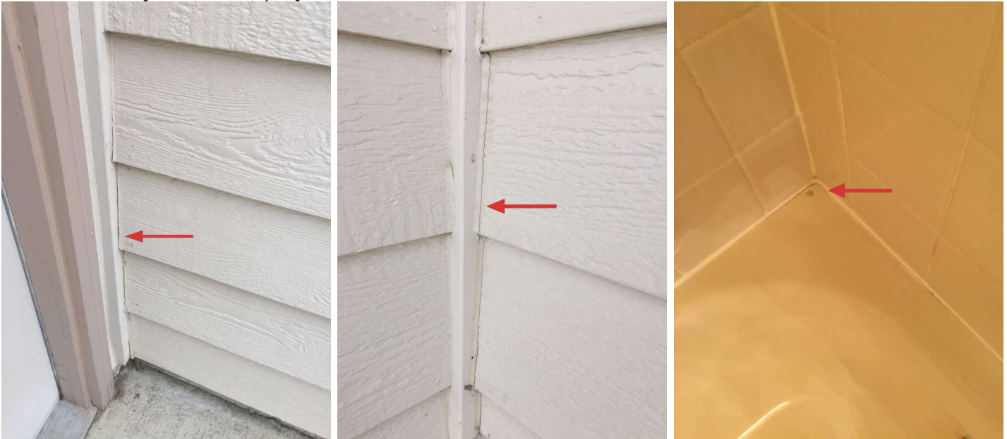
2nd Floor Bathroom Tub
