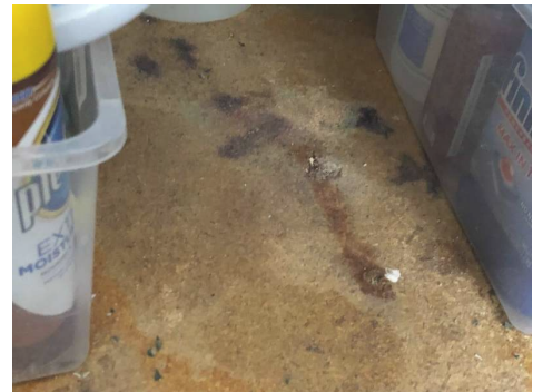
Moisture damaged cabinet floor.
