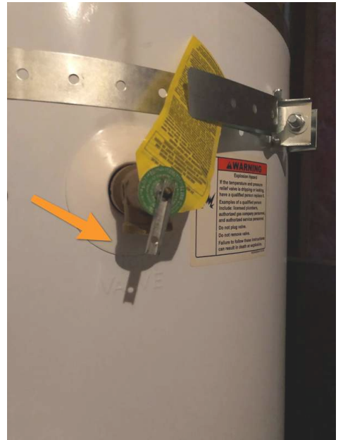
Missing discharge pipe here.
