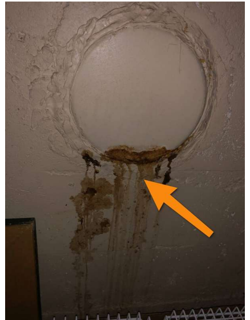
Previous moisture intrusion.
