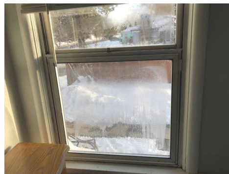
Seals blown between panes.
