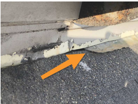
Flashing from sidewall over side entry roof stops short, it should be continuous across roof.
