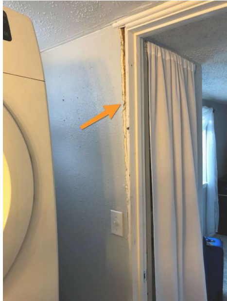
Missing door trim.
