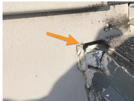
Kickout flashing missing here, with evidence of previous moisture exposure.
