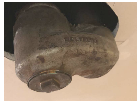
Drum trap below main bath. These are old school.
