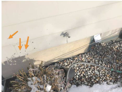
Various siding penetrations need sealed.
