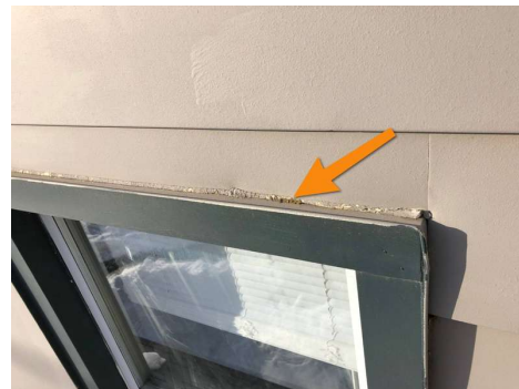
Caulk deterioration.
