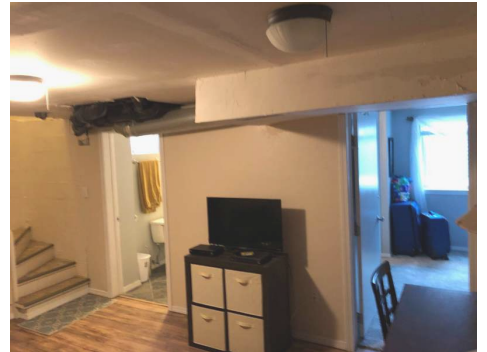
Basement ceiling drywall.
