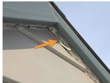
Failing caulk.
