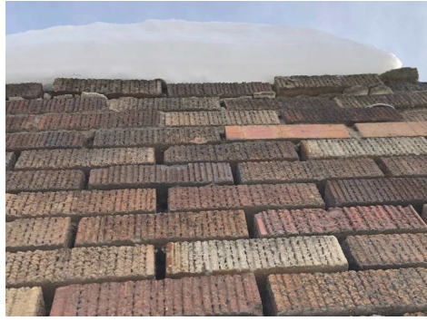
From the top down there are at least 13 courses of brick that need mortar repointed.
