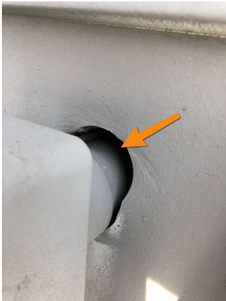
All penetrations like this one need to be sealed.
