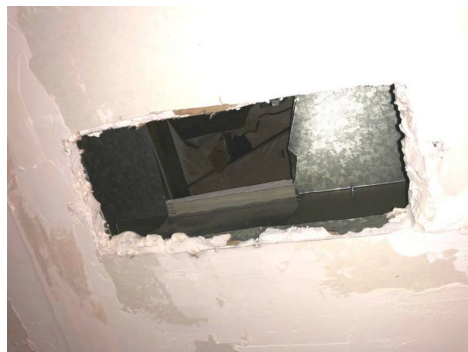
Open ducting above ceiling register.
