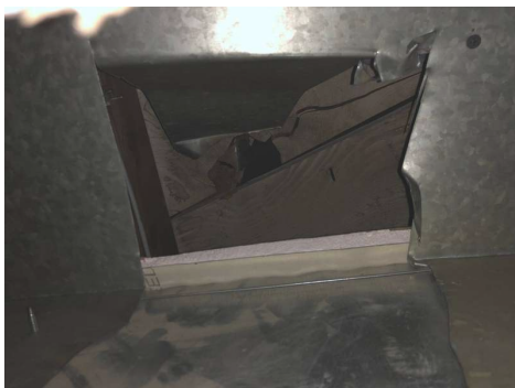
This HVAC trunk line has been cut open.
