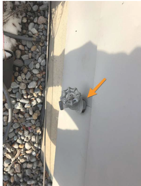
Seal here. Also this is not a frost free hose bib, so good idea to protect in winter, and/or replace in future.
