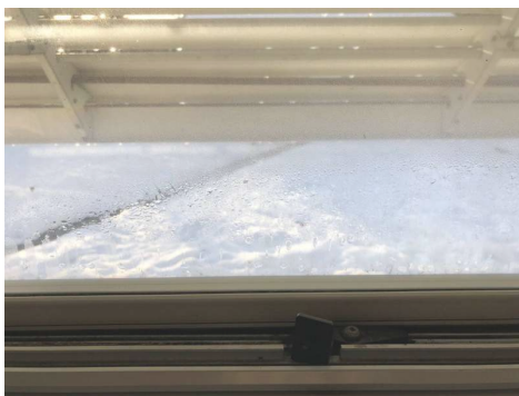
Condensation between window panes.
