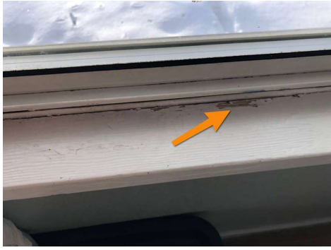
Paint failing.
