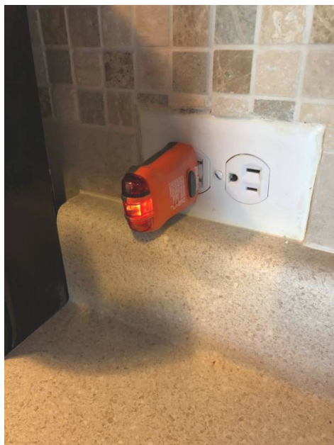
Open Ground/No GFCI.
