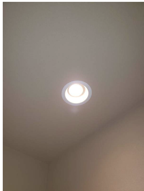
At shower enclosure.
