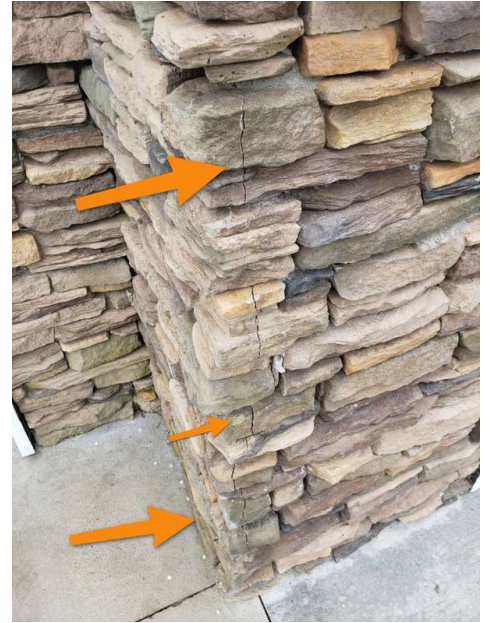
Cracking believed to be due to settlement. Correct to protect against moisture intrusion.
