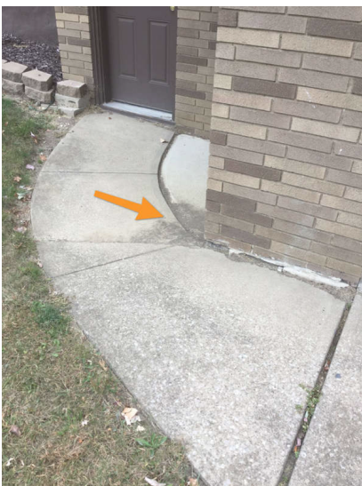
Dirt buildup from water runoff
