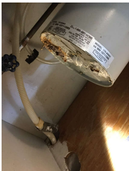
Bottom of unit is corroded and power is disconnected
