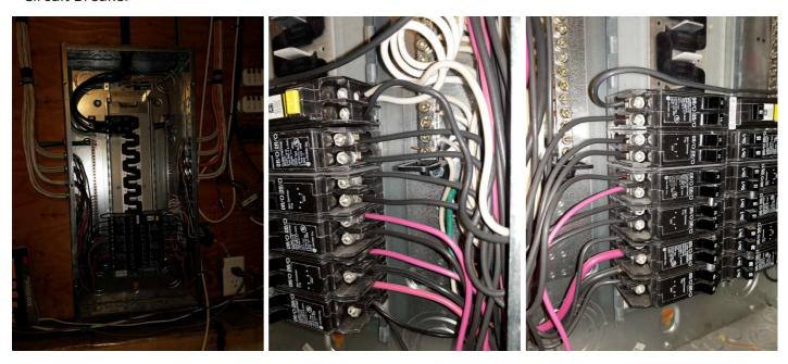
Branch Wiring Circuits, Breakers & Fuses: Wiring Method  $\,$  NMD  $\,90\,$
