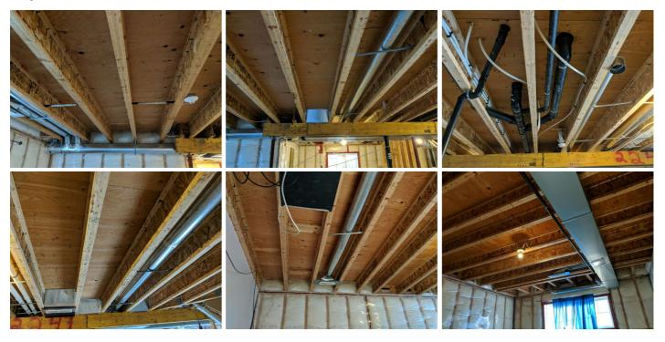
**Floor Structure: Material**Wood Beams, Wood I-Joists, Steel teleposts
