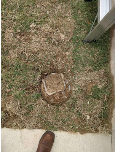
Location of Main Water Supply Valve : Main Level, Front Yard within 15ft of Street
