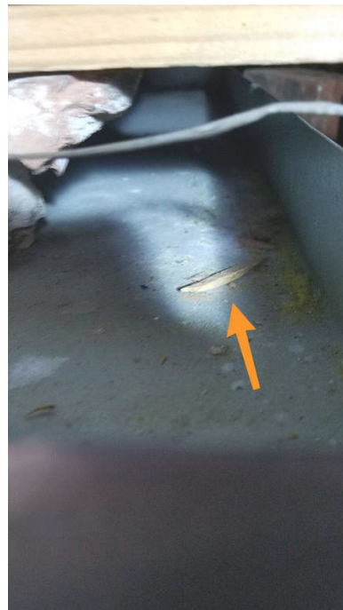
Attic, downstairs unit
