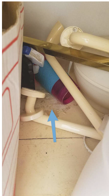
Upstairs Bathroom Left
