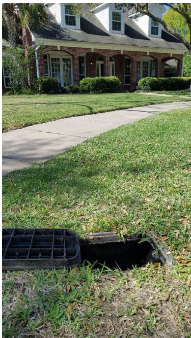
Location of Main Water Supply Shutoff Valve : Left side
