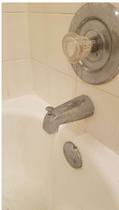
Upstairs Bathroom Left
