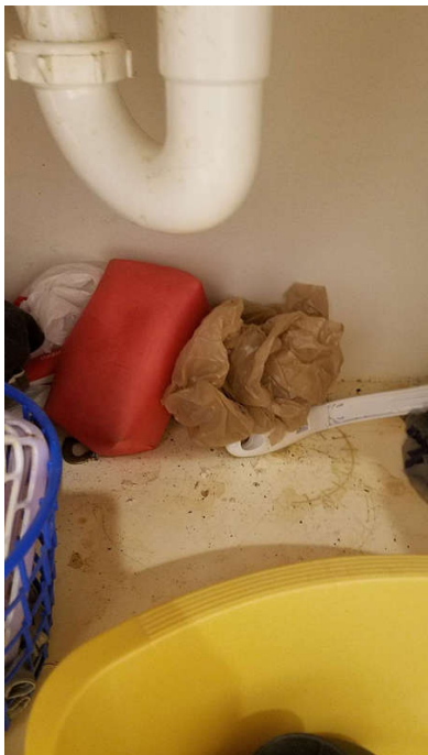
Upstairs Bathroom Left
