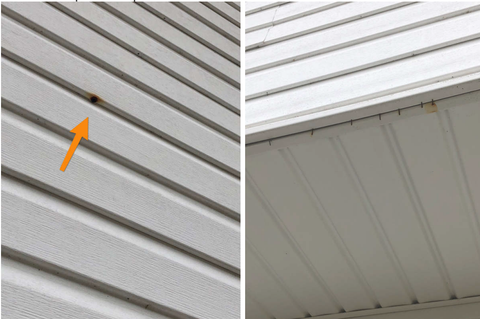
Non sealed screw exposed
