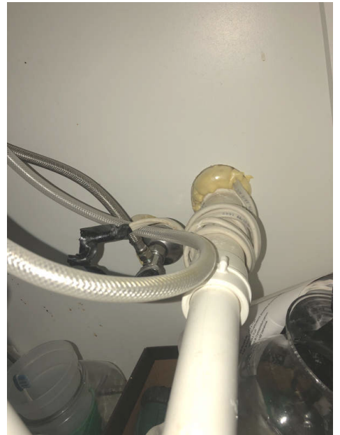
Wire taped off and in reach
