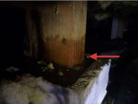
Splashback on support post from leak under utility room bathroom.
