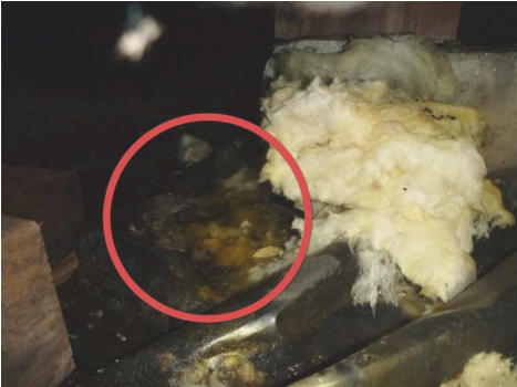
Ponding from leak under utility room bathroom.
