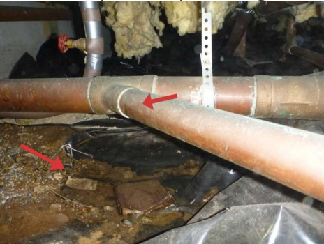
Leaking drain pipe with ponding on vapor barrier
