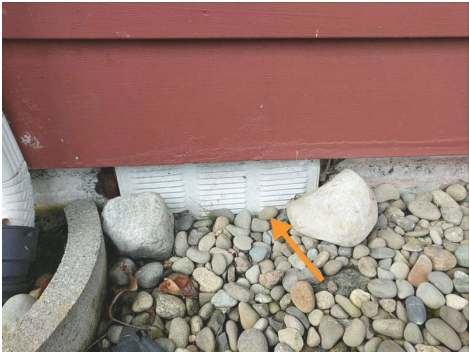
Foundation vents loosely held in place by rocks.
