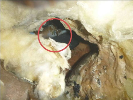
Leak in pipe under utility room bathroom
