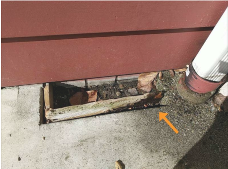
Vent located next to downspout drain and partially blocked by dirt.
