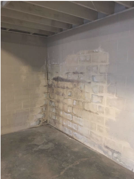
Right Rear Basement
