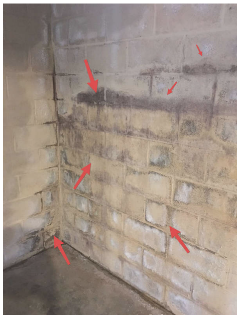
Right Rear Basement
