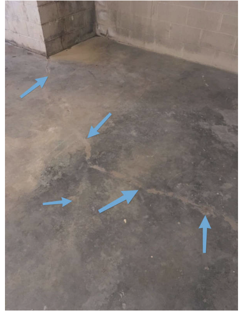
Right Rear Basement
