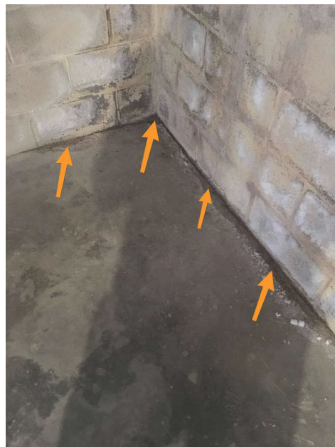
Rear Right Basement
