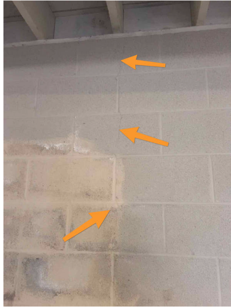
Right Rear Basement
