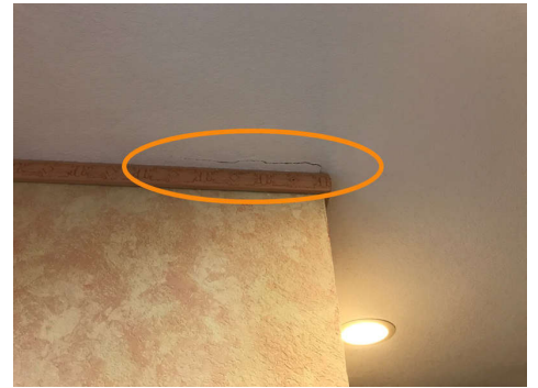
UNIT 3 South behind reception
