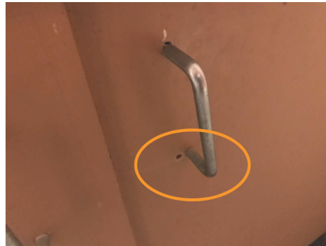
UNIT 2 main office Bathroom
