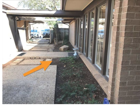
Unit 3 facing North
