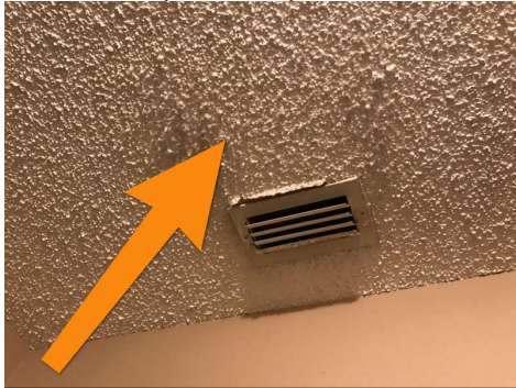
UNIT 1 West Bathroom
