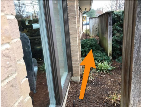
Unit 1 and Unit 4 facing North
