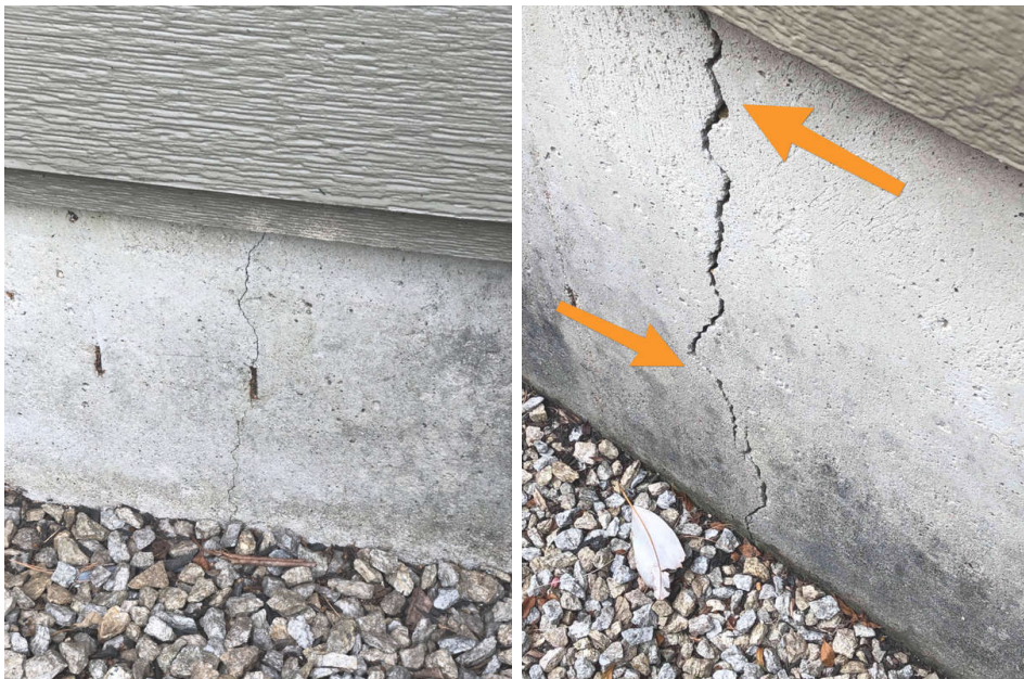
Left front, near elec meter
