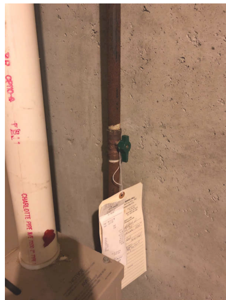
Unit A Shutoff
