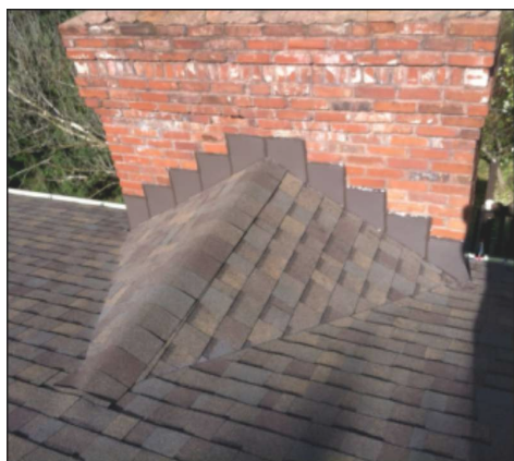
Example #1 of properly flashed cricket.
