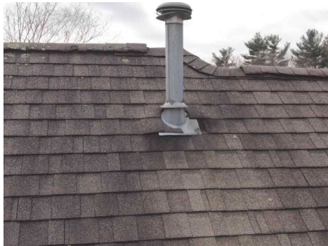
Example of properly flashed DWV Pipe.
