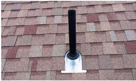
Example of properly flashed DWV Pipe.
