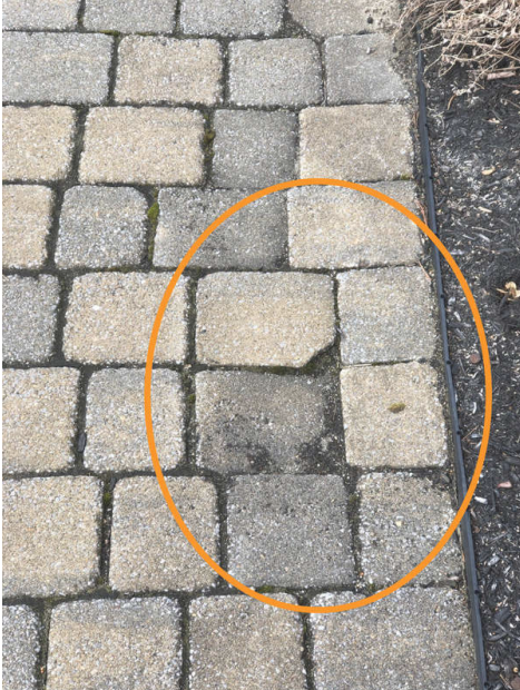
Pavers have sunk along stair tread
