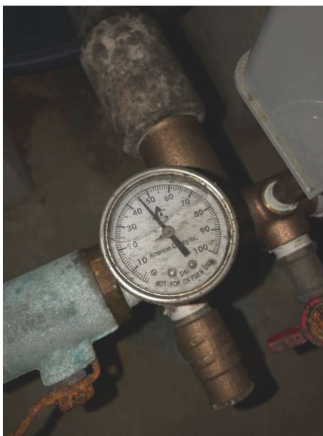
Main Water Pressure.
