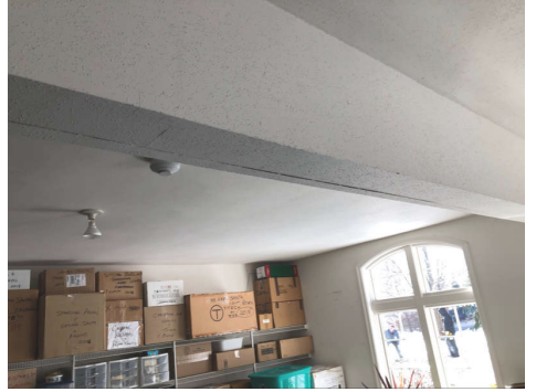
Corner bead pulling away
