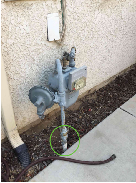
Main gas shut-off valve.
