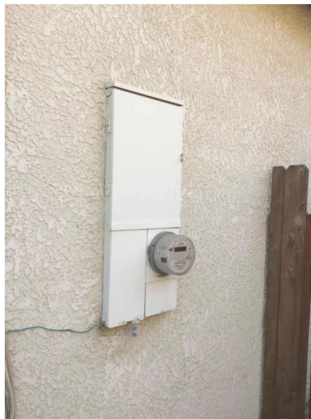
Electrical service panel.
