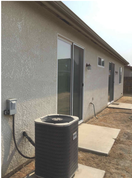
South side of building.
