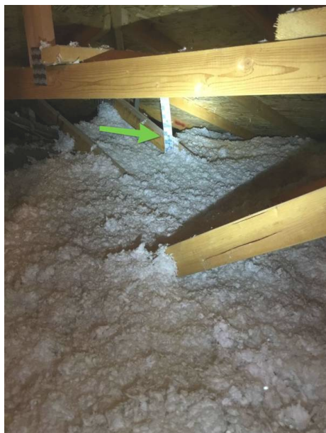
Insulation in attic.
