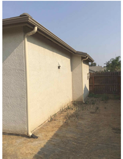
East side of building.
