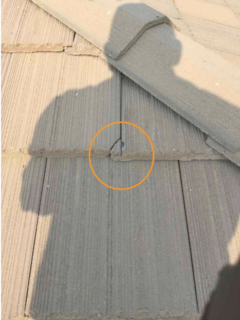
Condition observed at multiple locations.
