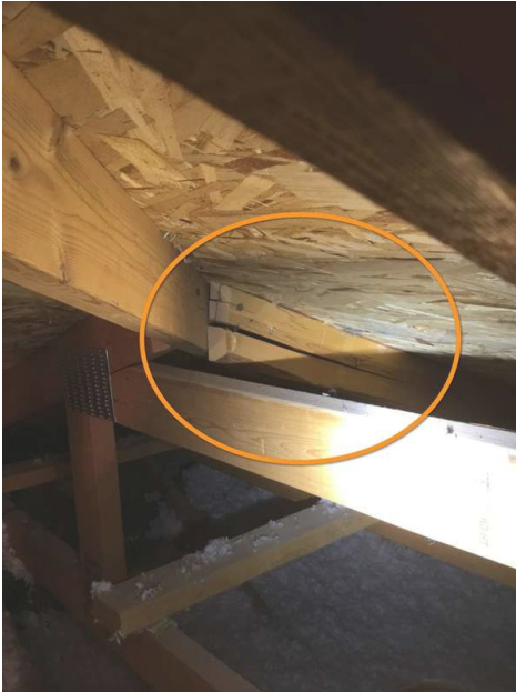
Near end of equipment platform looking Southwest.
