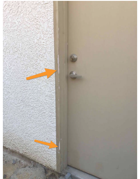
West side garage door trim.
