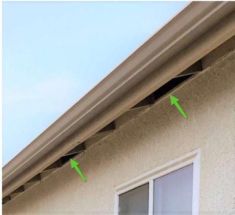
Soffit vents.
