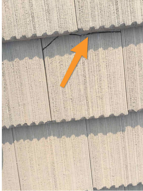
West side of garage roof.
