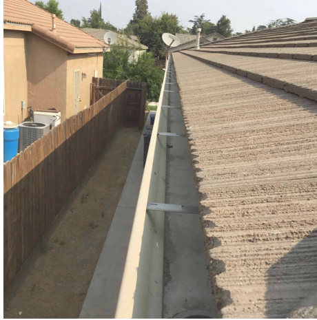
Representative sample of rain gutters.
