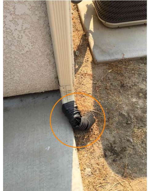
Southwest corner of building.
