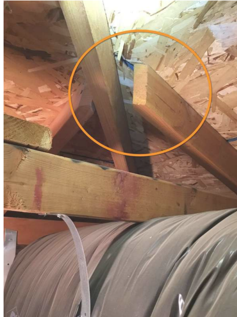
Near HVAC equipment looking North.
