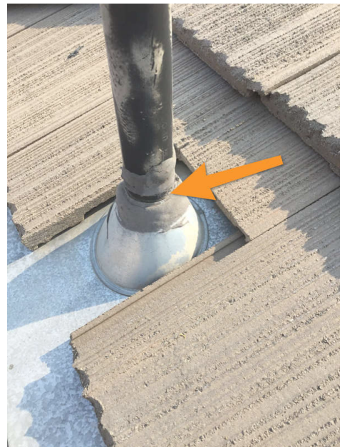
Condition observed at multiple locations.
