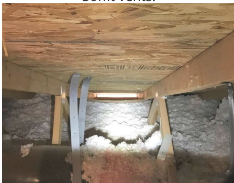
Soffit vent - attic view.
