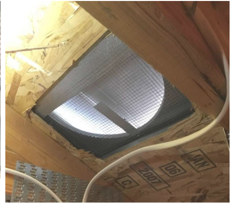
Off-ridge vent - attic view.
