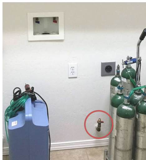
Gas shut-off valve for dryer.
