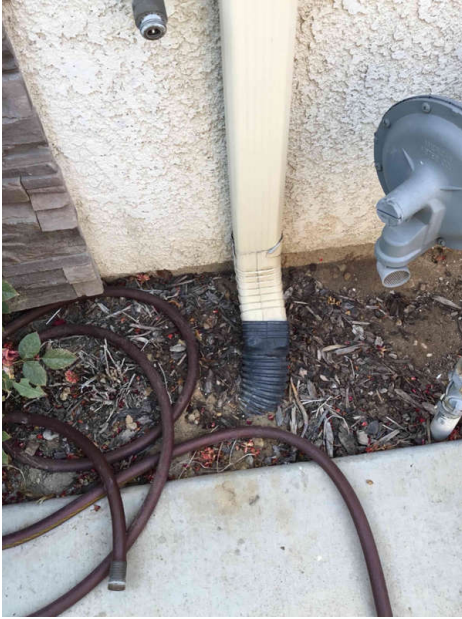
Representative sample of downspouts.
