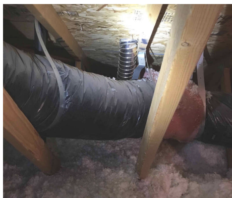
Insulated flexible HVAC ducts.
