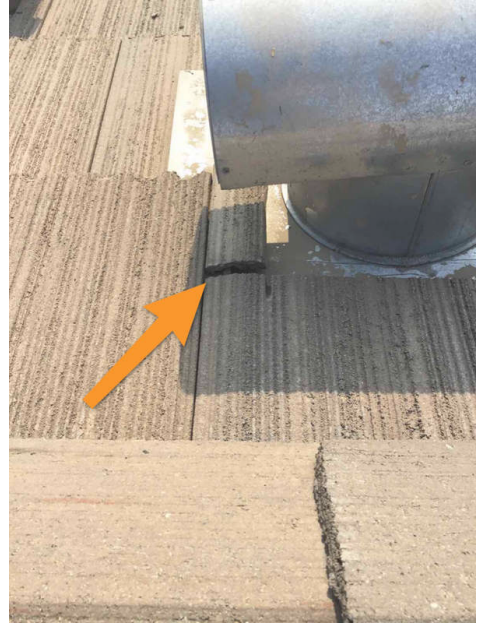
East side of garage roof at ridge.
