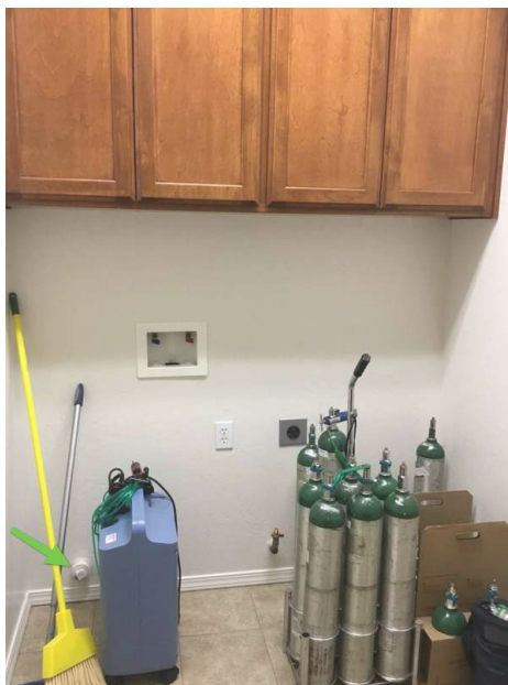
Laundry room on West wall.
