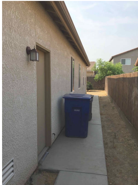
West side of building.
