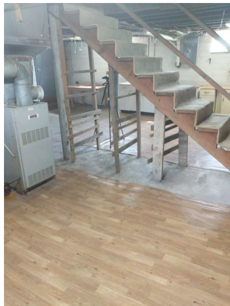
Basements & Crawlspace: Basement
