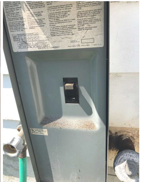
Main Shut Off
