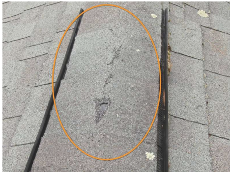
Shingle worn through
