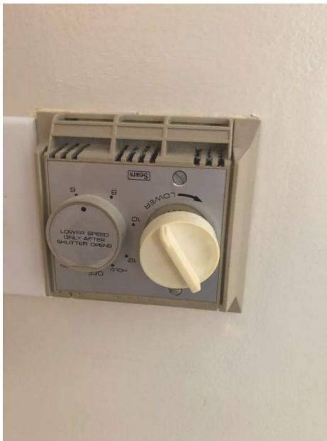
Whole House Fan Controls
