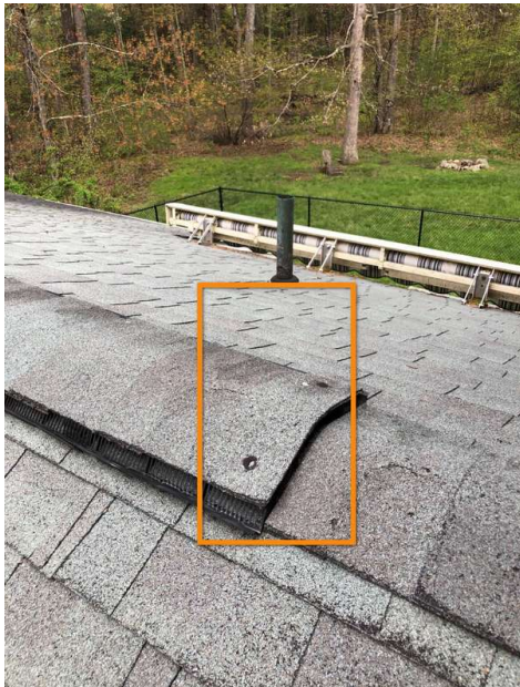
Cracking at ridge vent
