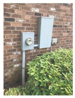
Main & Subpanels, Service & **Grounding, Main Overcurrent Device: Panel Capacity (Amp** Rating) 200 AMP
