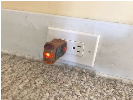
2nd Floor Hallway
