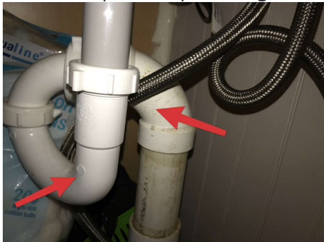
1st Floor Bathroom
