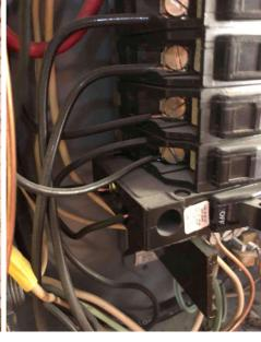
6.3.1 Branch Circuit Conductors
